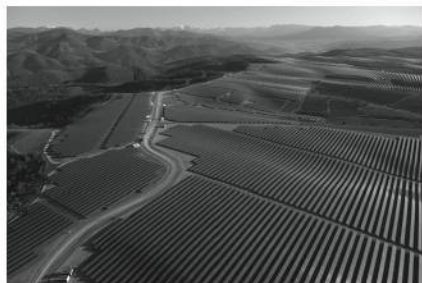
FIGURE 37.21 Les Mées solar farm in France comprises 113,000 solar panels, giving a peak power output of 100 MW.
