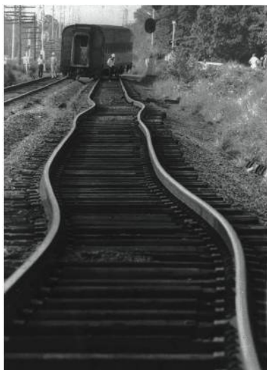
FIGURE 17.7 Thermal expansion distorted these tracks, causing a derailment. Expansion of long structures like this is best described using the coefficient of linear expansion.
