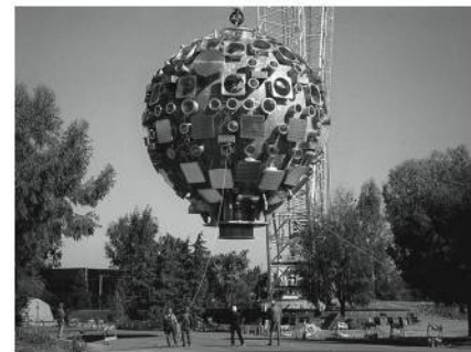
FIGURE 23.17 The NIF target chamber, shown during installation (Passage Problems 70–73)
